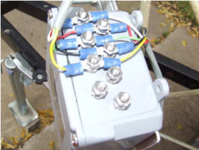
Note the installation of the leads
